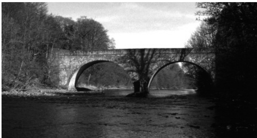
Figure 3. The Teith Bridge, south of Doune.
