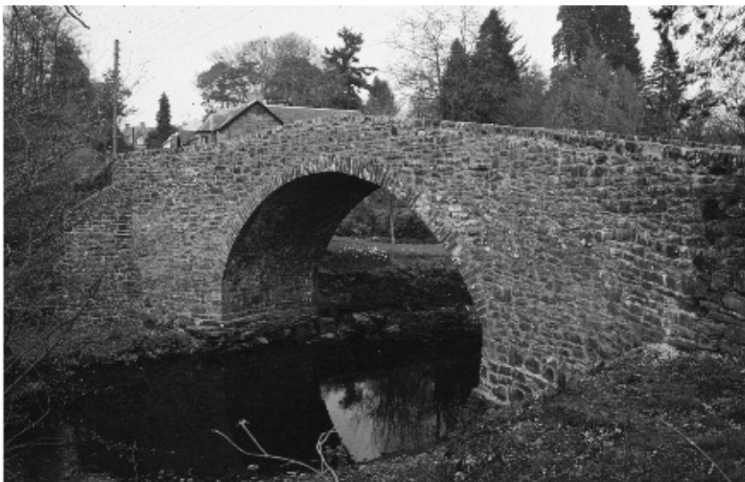
Figure 2. Bridge over the Ardoch Burn at Doune.
