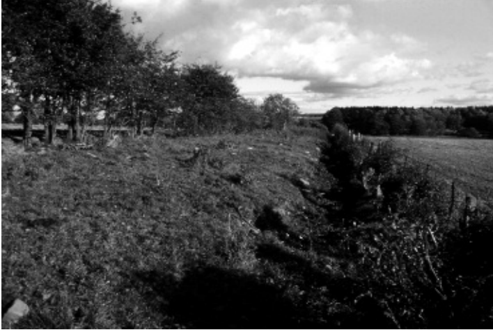
Figure 3. Roman road, near Arduvie Farm, on Gask Ridge, showing the raised roadway ( agger ).
