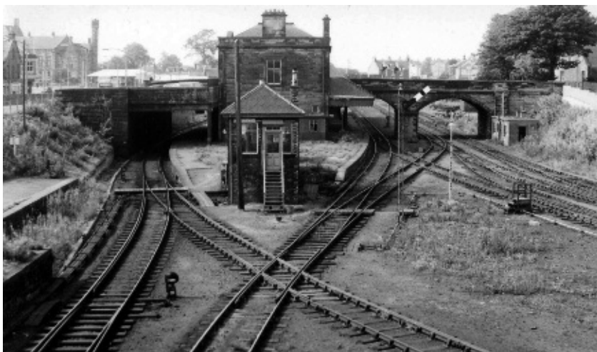
Figure 3. Old Alloa station looking west. Alloa East Signal Box controlled the junction to the Devon Valley Line which leaves on the right. The main line to Dunfermline leaves Alloa on the lines out of the bottom of the picture while trains headed for Stirling had to pass through the station. At one time five signal boxes controlled the line between Stirling and Alloa. The entire new railway line is controlled by a signalman in Stirling Middle Signal Box watching over the trains using CCTV and other safety devices. ( Picture: Clackmannanshire Council Library Services. )
