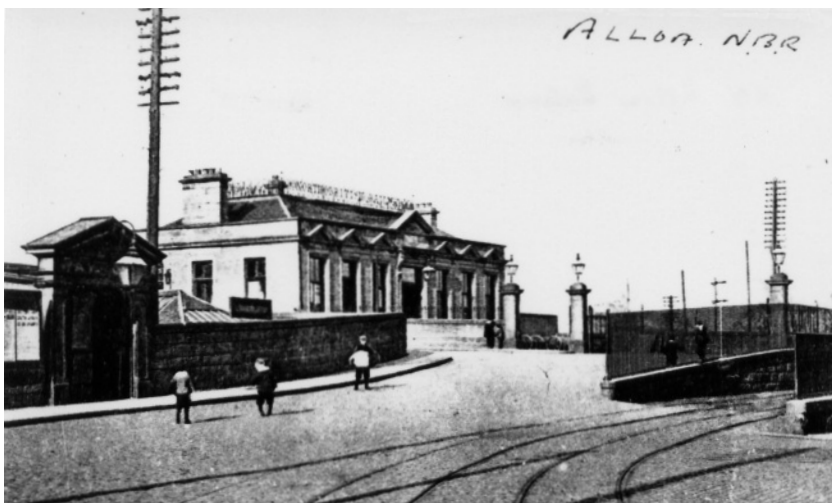
Figure 1. Alloa Station, c 1910. The station was rebuilt in 1885 by the North British Railway Company. It put right all the inconveniences and dangers of the original station. The remains of the derelict station were finally demolished in 1984. The new station was built a few hundred yards to the east of this building located on the old Alloa Brewery site. The new station has one platform and the building is unmanned. (Picture: Clackmannanshire Council Library Services.)
