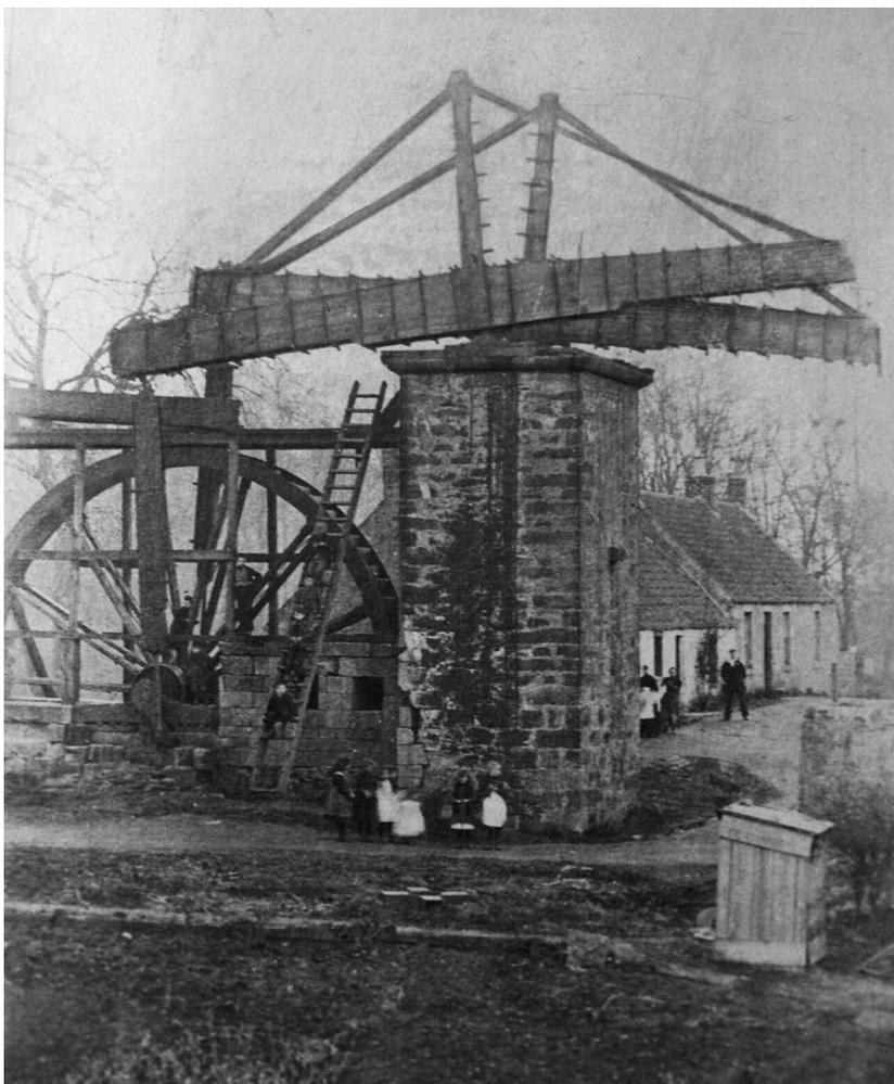
Figure 7. Water Powered Pumping Engine at the Old Watermill Pit
