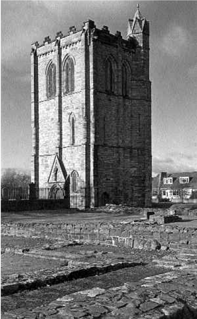
Figure 5 Cambuskenneth Abbey, Bell Tower, foundations of cloister and nave. (L. Main)
