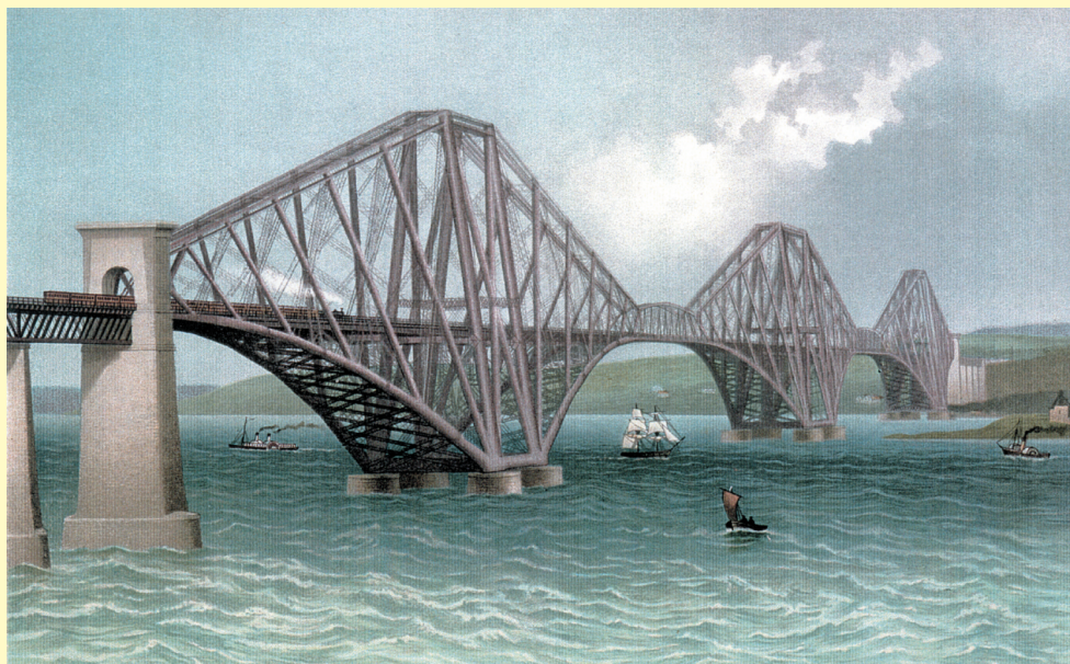
Forth Rail Bridge 1892.
