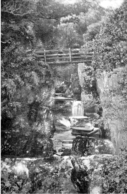
Figure 16 Bracklinn Falls Bridge.
