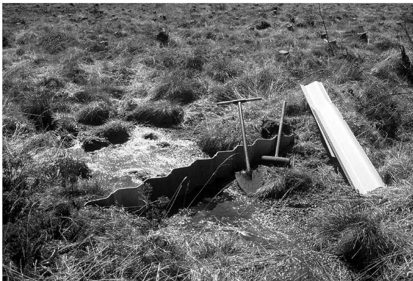
Figure 2 – A ditch dammed with recycled plastic piling installed to slow water flow off the moss.
