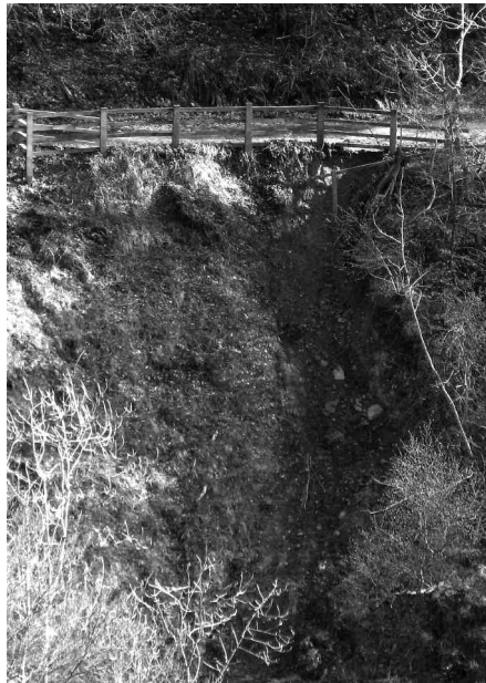
Figure 10. View of the scar taken from across the valley. This shows how blocks of unconsolidated till rapidly break up into debris flows on the steep slopes below the road (slopes exceed 35^{\circ} in many places).
