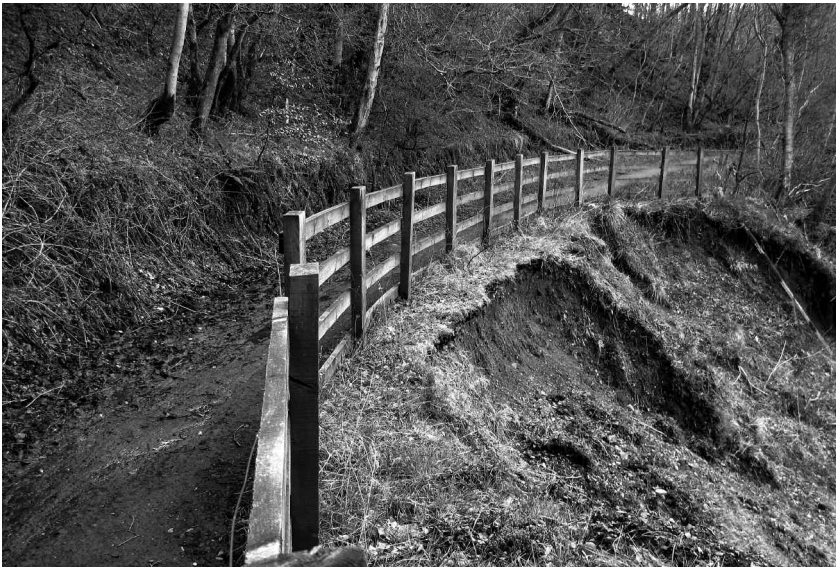
Figure 8. State of the head scar of the main landslide in April 2009. Patchy re-vegetation can be seen but, in places the slide has been re-activated leading to small-scale slides and flows.
