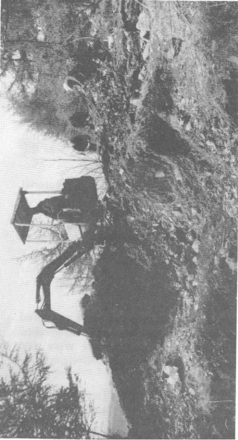
Sorting and selecting material excavated
