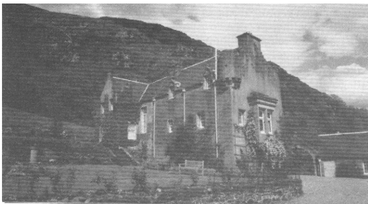
'The Blair', Blairlogie Castle - 1543 tower-house in foreground, oriel window added in 1890's.
