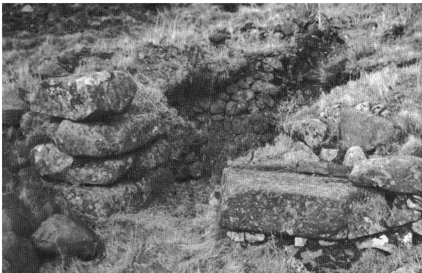
Plate 5. Well-preserved lime-kiln at foot of Sauchie Crag. This is situated on the platform visible on lower left corner of Plate 4.
