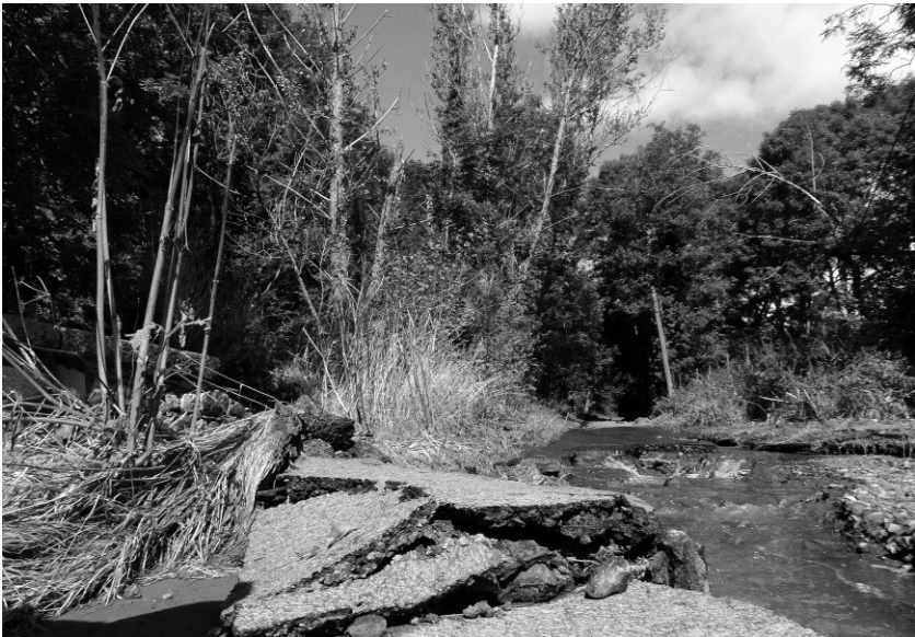
Figure 3b. Tarmac forced into the side of the road by water pressure at location of 3a.
