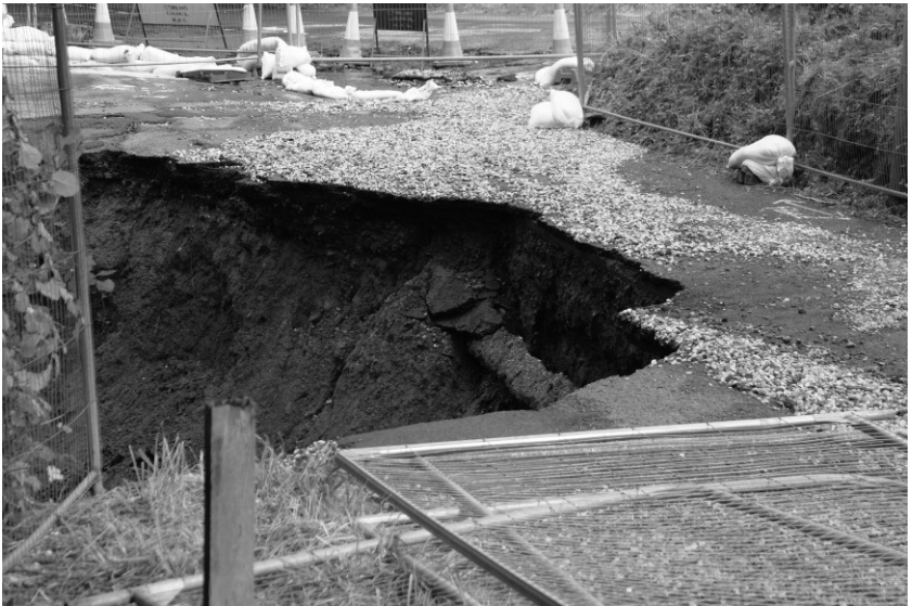
Figure 1b. Gully-head at location of 1a, showing exposure of service conduits and road closure.
