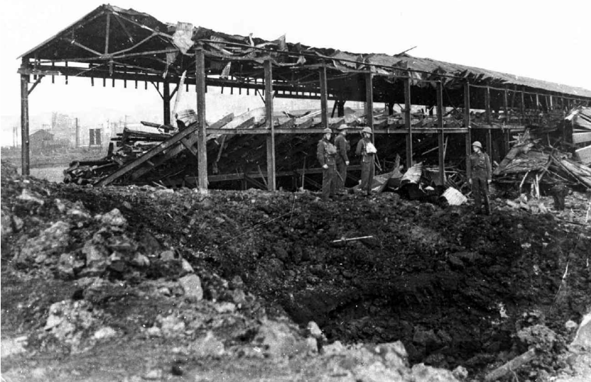
Figure 2. The grandstand at Forthbank after the bomb, dropped by a German plane, landed on it in the early hours of 20 th July 1940 (with kind permission of The Smith Art Gallery and Museum).
