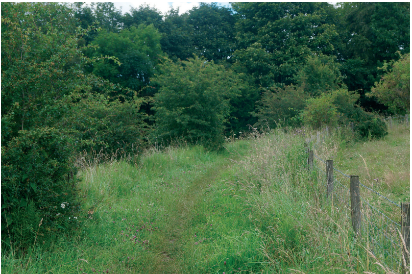
Plate 1b. The remains of one of the two piers on the River Black Devon.
