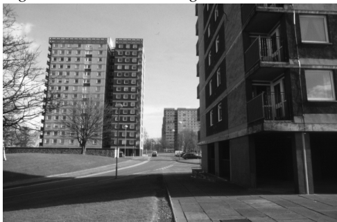
Figure 12. Callendar Park high rise flats.
