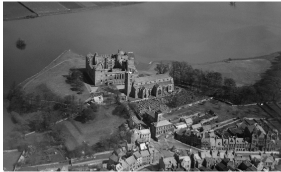
Figure 2. Aerial view of Linlithgow Palace. ©HES SPWO 17716.
