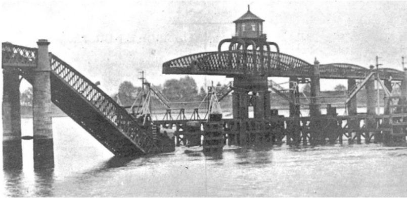
Figure 16. Damage caused by collision with a steamer in 1904.
