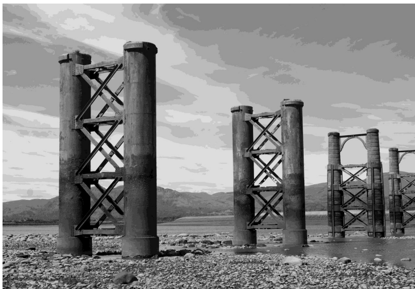
Figure 19. Replacement metal piers.
