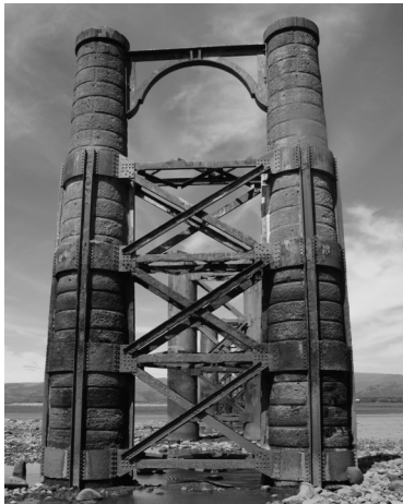
Figure 18. Remains of metal and stone piers.
