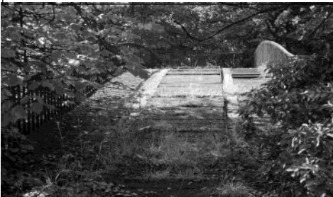
Figure 6. Cambus Bridge Deck
