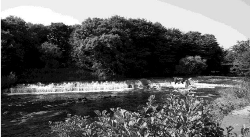
Figure 13. The “V”-shaped weir across the river Devon at Cambus.
