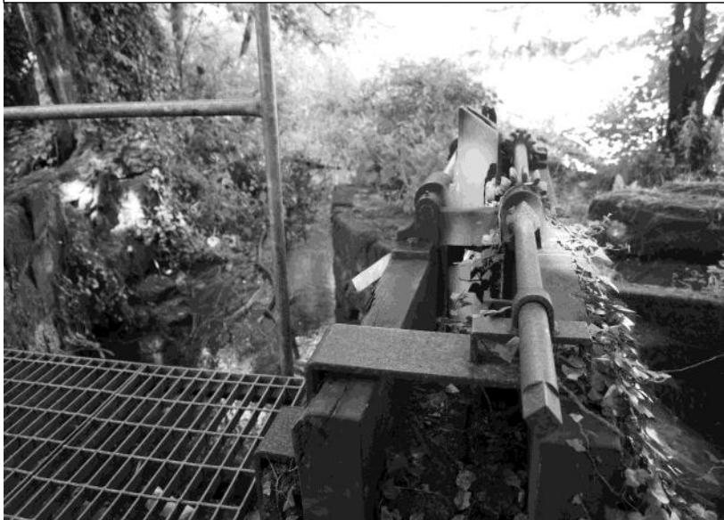
Figure 14. The Sawmill lade and sluice.
